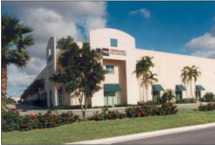
"Tilt-Wall" construction warehouse with facade scaling elements and articulated entry points.
