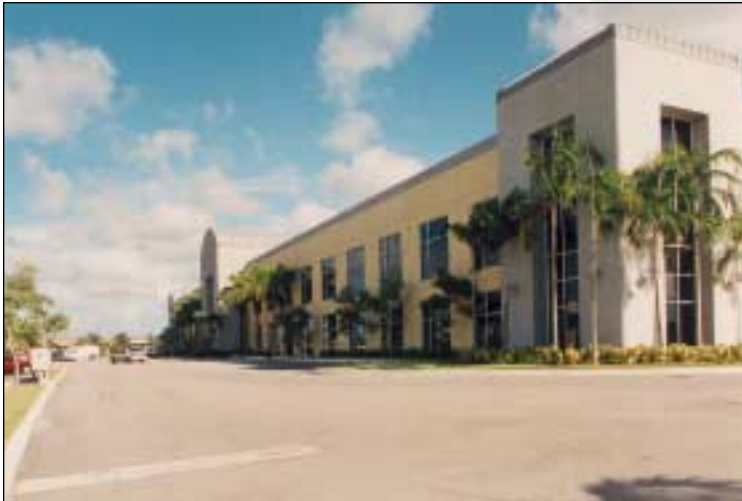
A renovation of an existing warehouse using a new "Tilt Wall" skin and entry tower elements.
