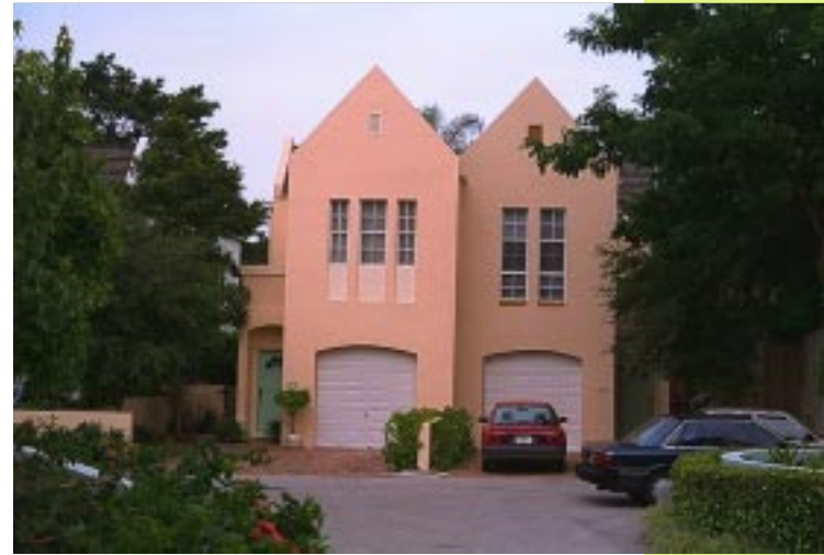
Duplex units sited as an auto-centered cluster. Units could be improved by making the entry points a dominant feature of the facade design.
