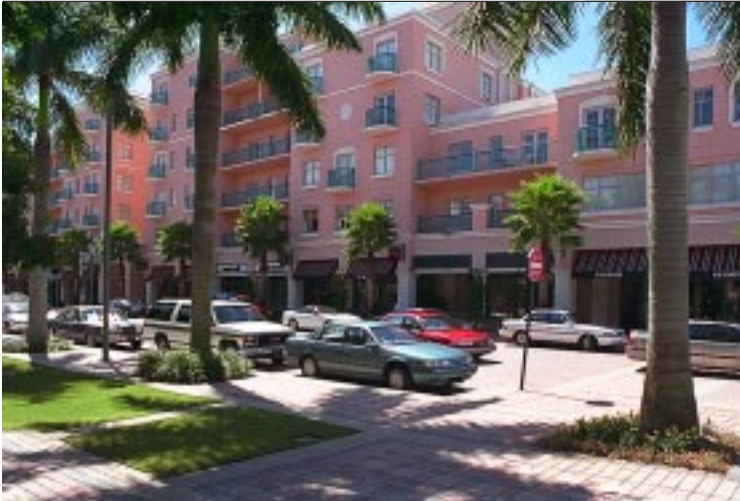
Owners of these luxury apartments above this retail street can easily enjoy the amenities provided.
