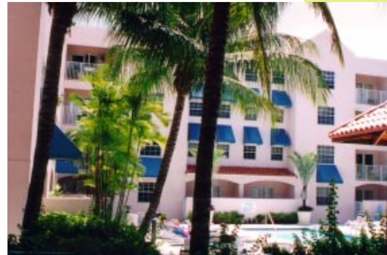
A simple pipe frame awnings adds shade, detail and color to this facade.
