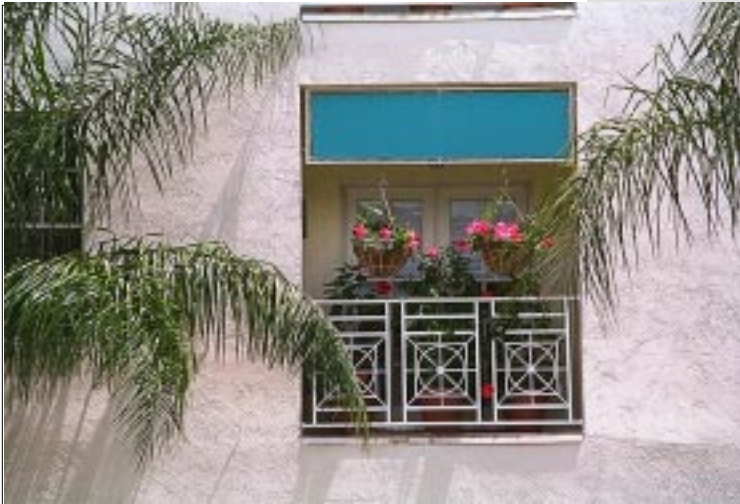
Balconies built into the "building mass" provide greater privacy than balconies "hung" off the facade.
