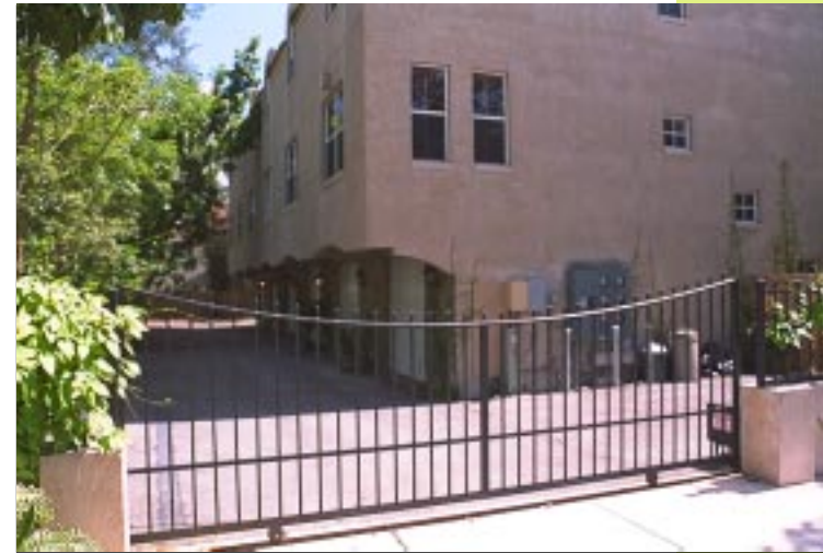
Garage entries and utilities grouped together and accessed off a secondary street.
