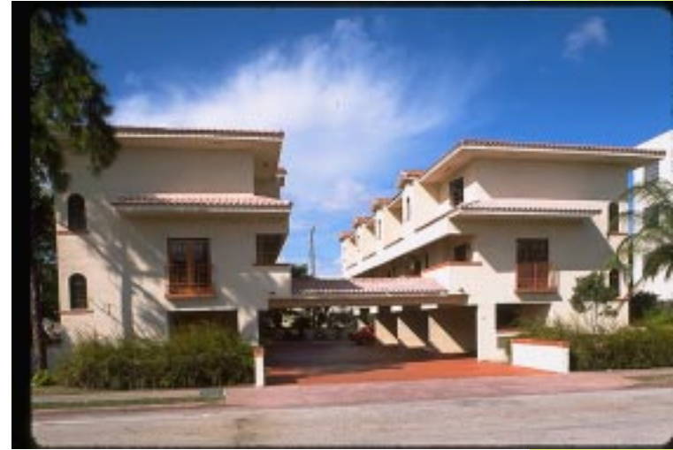
A typical "six pack" townhouse configuration which has parking underneath. A single loaded bar building sited perpendicular to the street with parking underneath is a good design type for a building with only a few units.
