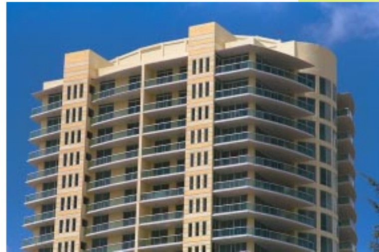
Towers are encouraged to have an interesting "terminal element" to add to the skyline.
