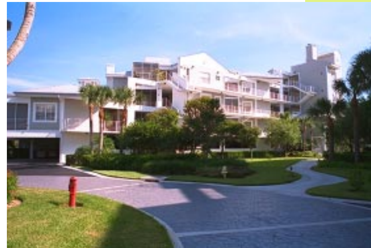
Units step up from one to five stories to lessen the impact of the building on the surrounding area.
