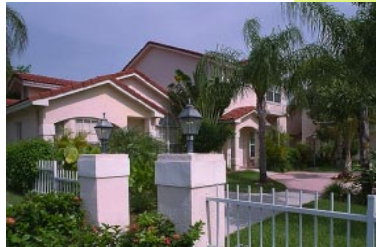
Houses sited around a pedestrian garden space.
