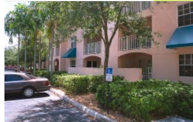
Private ground level patios off the parking are defined by "garden walls" and plantings
