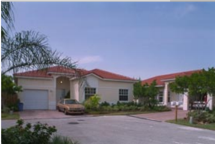
Careful overlapping of unit footprints minimizes blank walls and provides enclosure for entries.
