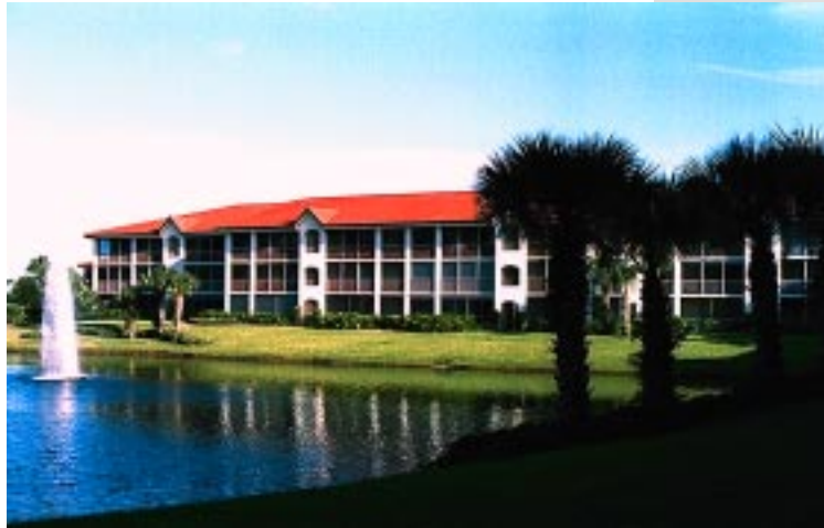
A common building type which works well for multifamily units is a single loaded "bar" building with intra-building entry towers. Screened balconies and porches provide private outdoor space.
