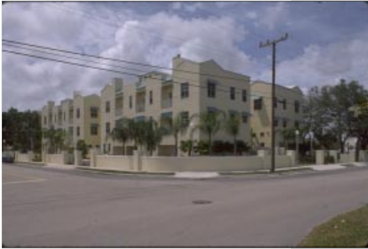
High density "urban" townhouse units which have parking and entries off the street.
