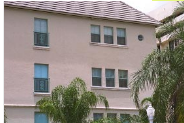
Cast stone sills, metal railings and the decorative round window on this facade provide an acceptable alternative to the required six inch wide trim on all window and door openings.
