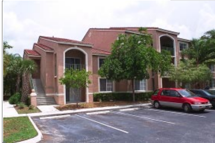
Individual units are expressed in the changes in the roof plane of this building.
