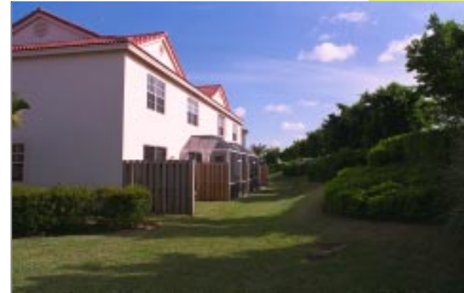
These units include small screen enclosures located along the street buffer.
