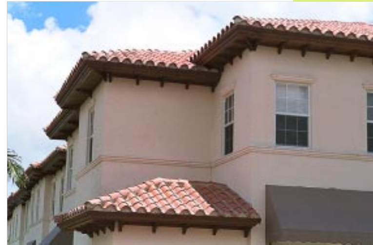
Multiple roof planes and a wide well detailed overhang make this unit interesting to look at.
