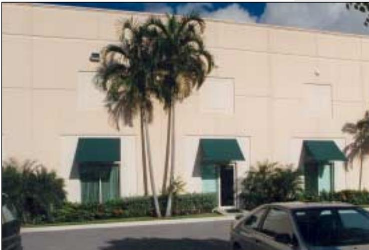
Wall panels, windows with awnings and plantings help scale this "Tilt Wall" warehouse.
