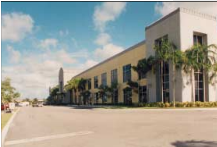
A renovation of an existing warehouse using a new "Tilt Wall" skin and entry tower elements.
