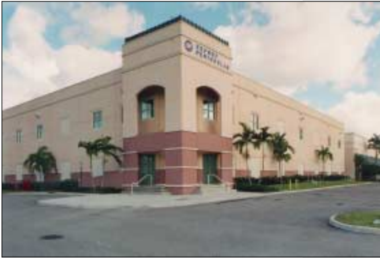
Articulation of the base with stucco relief and a secondary building color help scale this warehouse.
