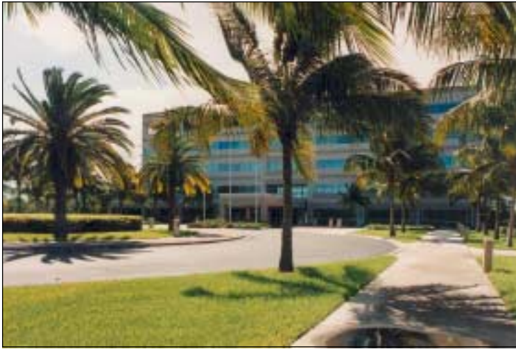
A "signature" entrance with a well developed pedestrian connection to the parking lot.
