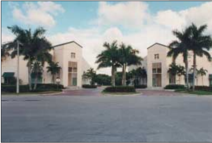
Twin tower entry elements located at the corners add interest, and share an vehicular entry drive.
