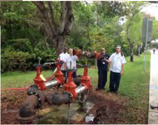
Installing a new Backflow Preventer Assembly for backflow protection
