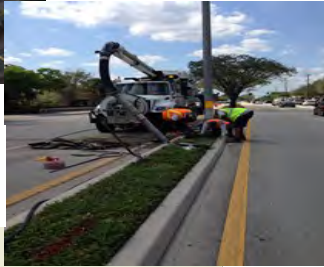
Service line leak repair on Sample Rd.
