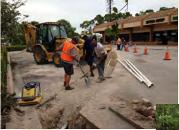
Installing a new Backflow Preventer Assembly for backflow protection
