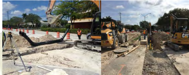
Raw Water Well Field Rehabilitation
