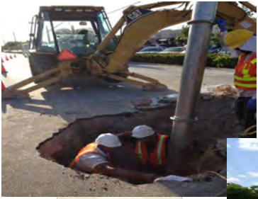
12" water main break repair on Sample Rd.
